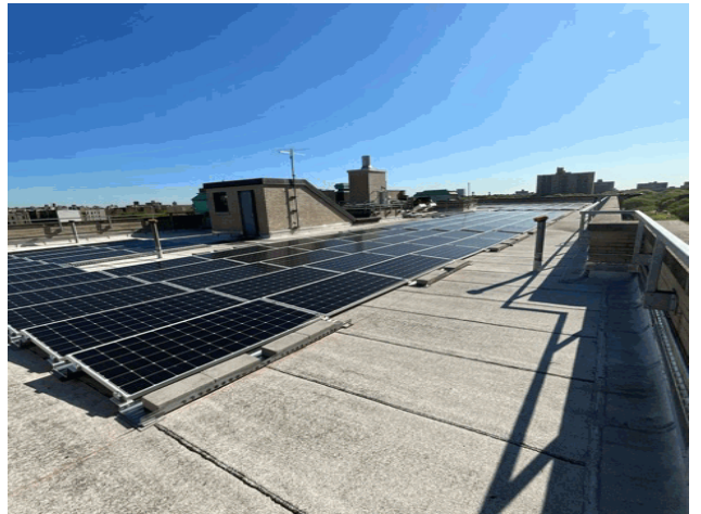
Roof 1 - East view
