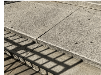
Facade A at Exit 8
