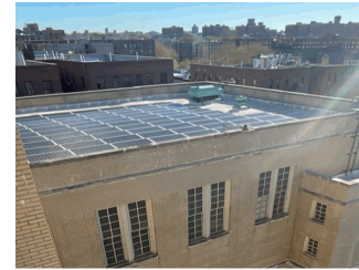
Roof 2 at Facade D
