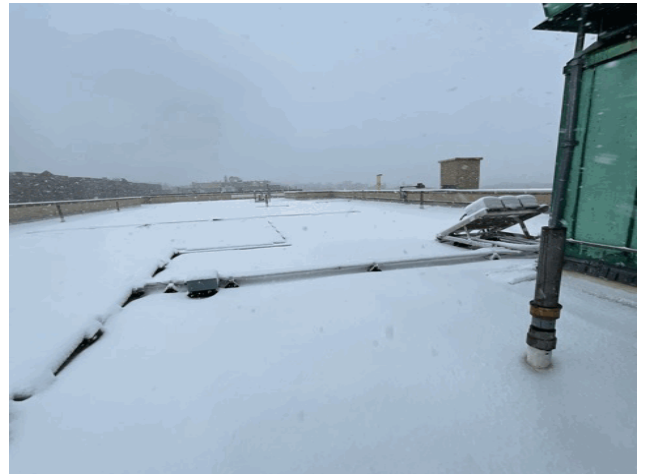
Roof 1 - Northeast View
