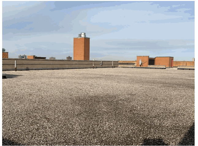
Roof 1 - Northwest View
