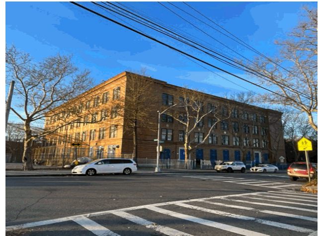
Corner of Mace Avenue and Willamsbridge Road - Northeast View
