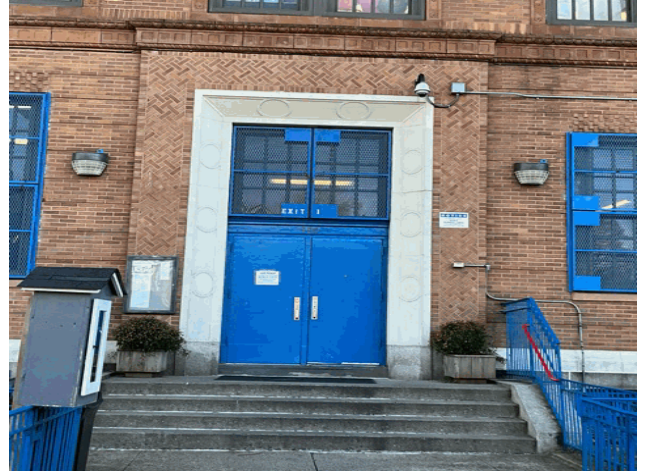
Facade A - Mace Avenue
