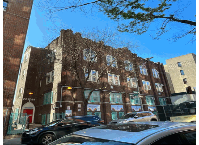
Sheridan Avenue - Northwest View
