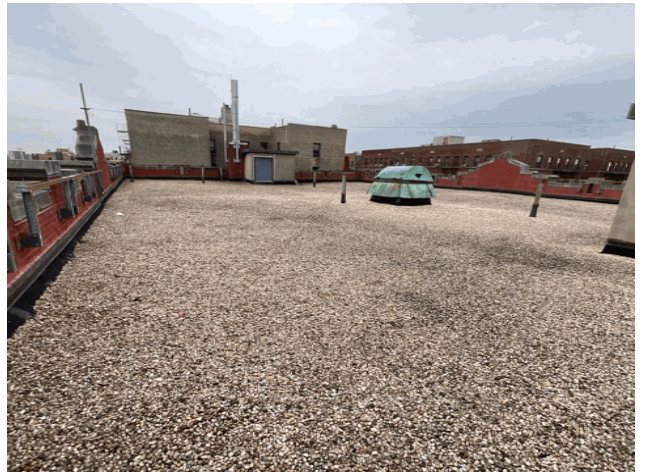
Roof 1 - Southwest View
