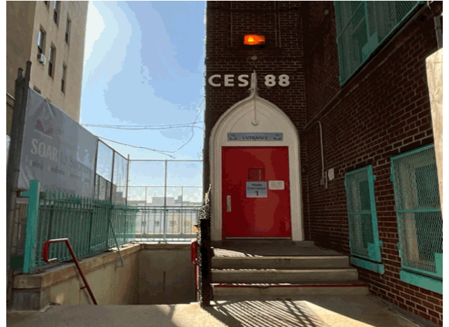
Facade A - Sheridan Avenue
