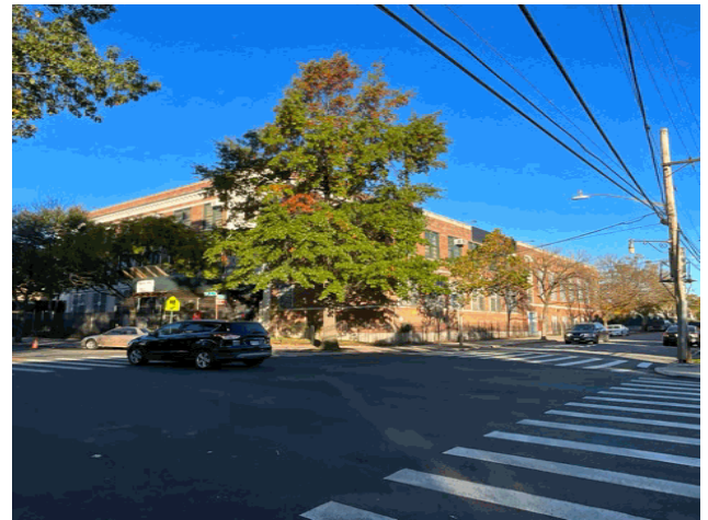
Corner of Bussing Avenue and Edson Avenue - Southeast View
