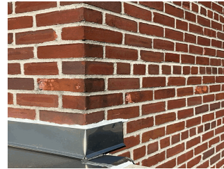
Roof 1 - Chimney CH1
