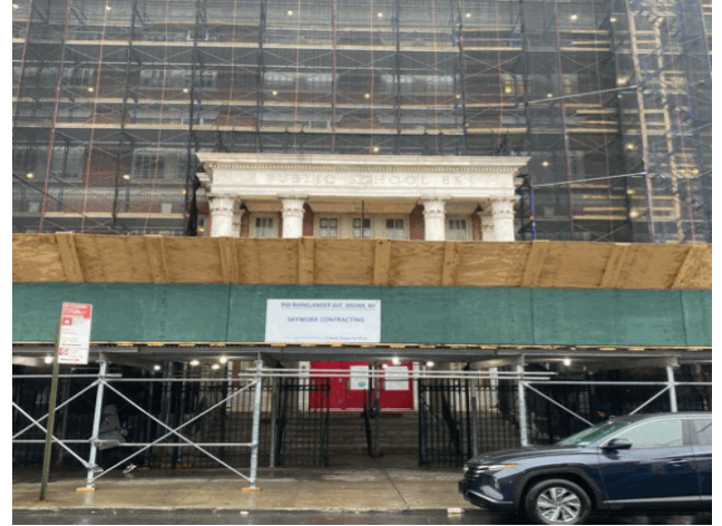
Facade A - Rhineland Avenue
