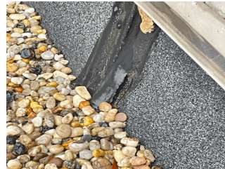
Roof 1 - Facade A
