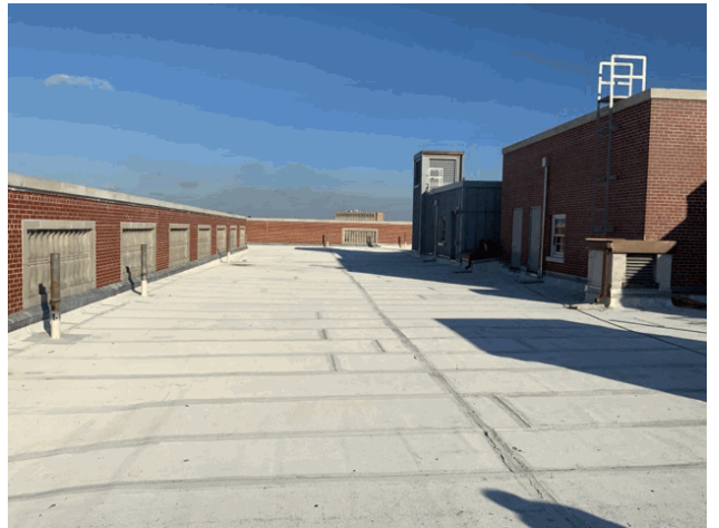
Main Roof - North View
