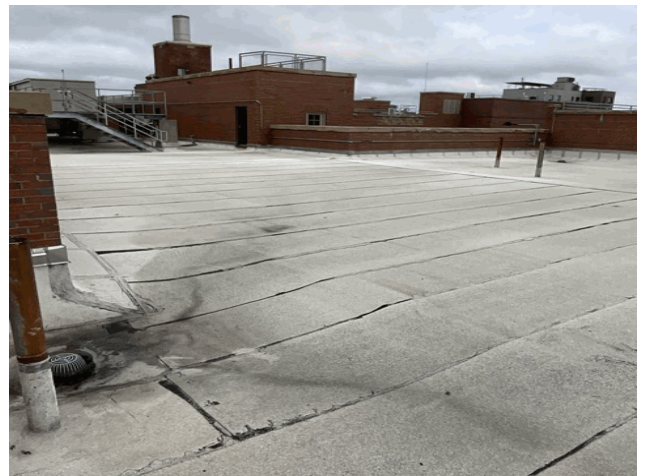
Roof 4 - North view
