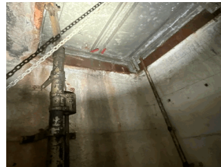
Ash Hoist Vault
