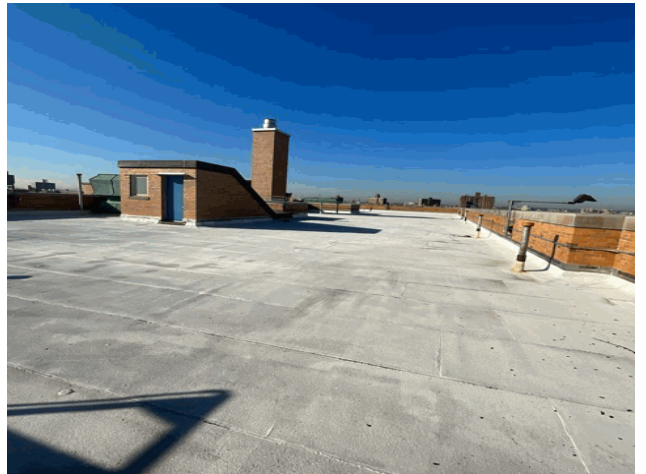
Roof1 - Southwest View
