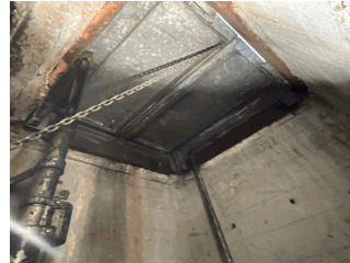
Ash Hoist Vault
