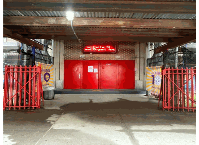
Facade A - Faile Street
