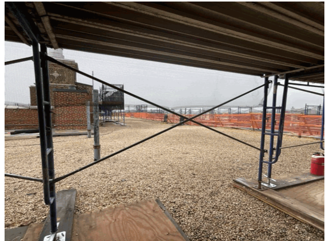
Roof 1 - South View
