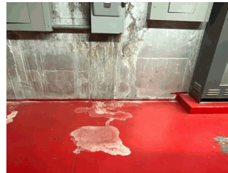
Electrical Panel Room
