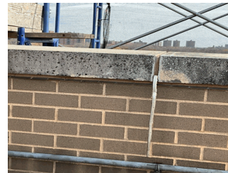
Roof 1 - Facade C
