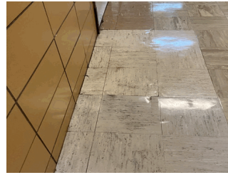
Corridor near Room 320
