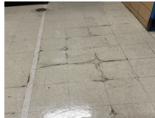
Corridor near Room 175
