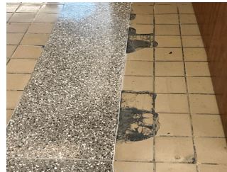
Main Entrance Lobby
