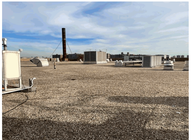
Roof 1 - North view
