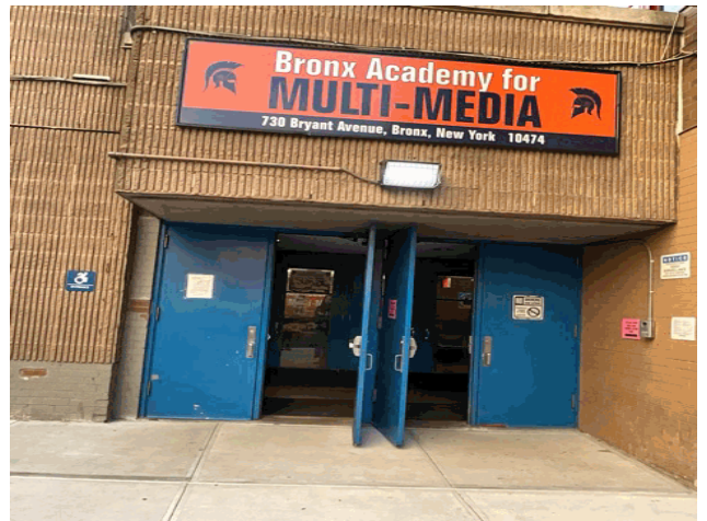
Facade A - Bryant Avenue
