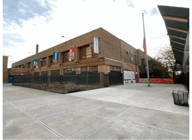
Bryant Avenue - Southwest View
