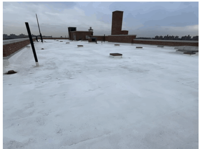
Roof 1 - Southwest View
