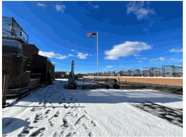
Roof 1 - South View
