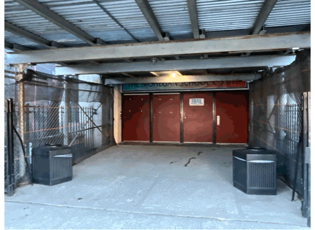
Facade A - Mohegan Avenue
