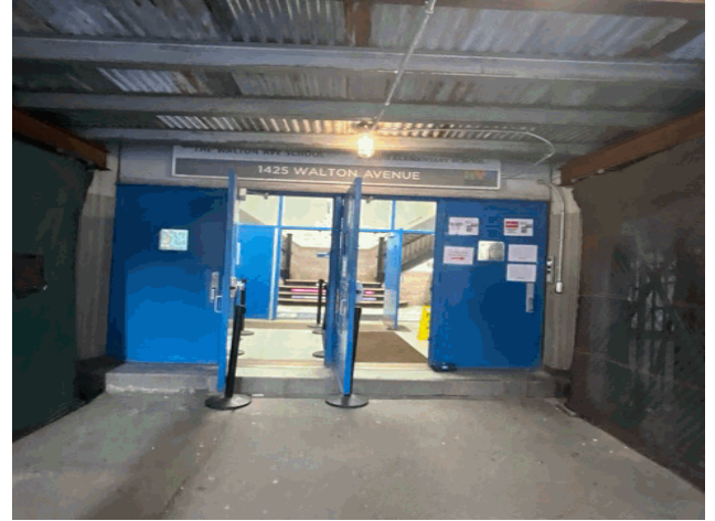
Facade A - Walton Avenue
