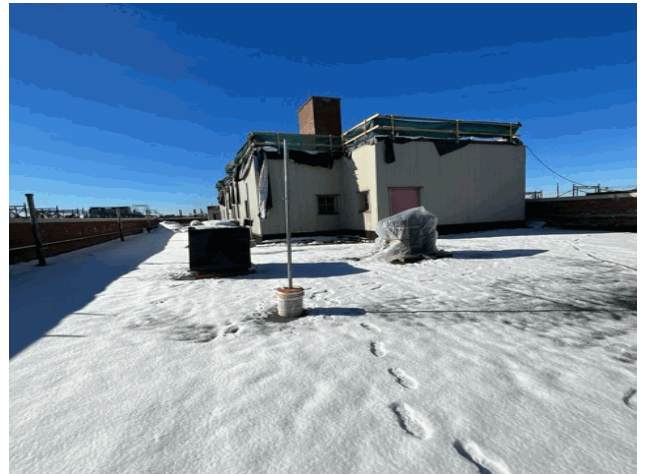
Roof 1 - North view
