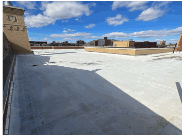
Roof 1 - Northwest View
