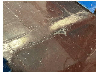
Corridor near Room 303
