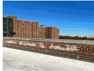
Roof 1 - Facade A
