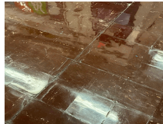
Corridor near Room 411
