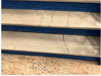
Main Entrance Lobby
