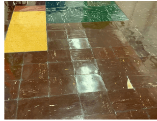
Corridor near Room 411
