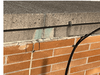
Roof 1 - Facade C
