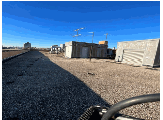
Roof 1 - North View
