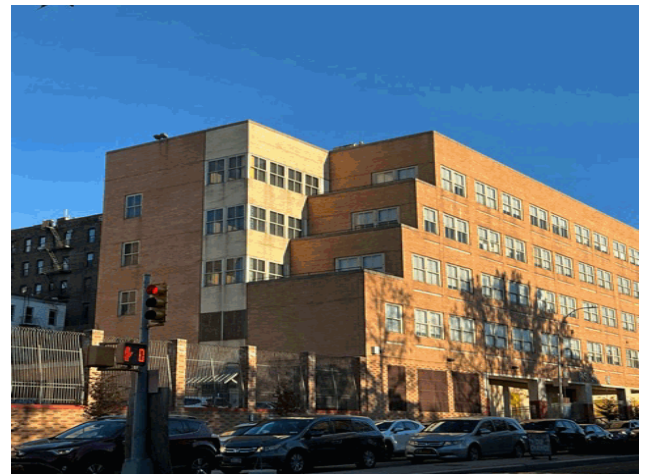
Corner of Webster Avenue and East 195th Street- South View
