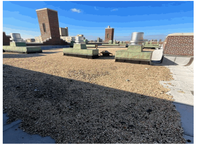
Roof 1 - West View
