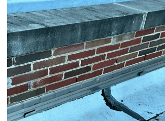
Roof 2 - Facade V
