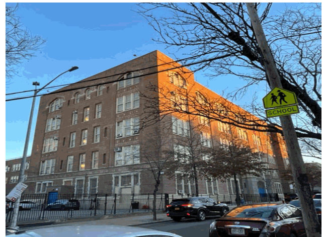
Kelly Street - Northeast View
