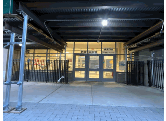
Facade B - Briggs Avenue
