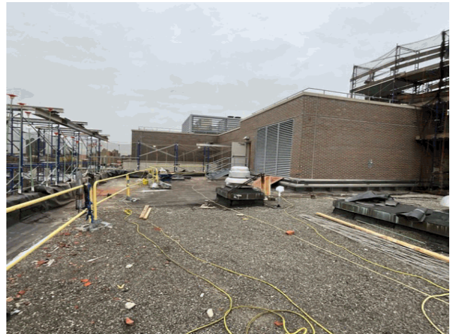
Roof 1 - Northeast View
