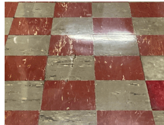
Corridor near Room 104A
