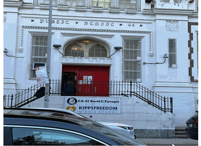
Facade A - Prospect Avenue
