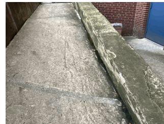
Areaway AW1 - Kitchen Ramp
