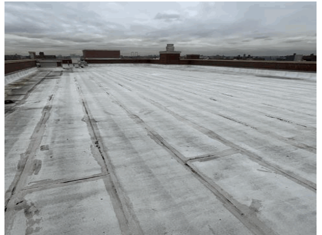
Roof 1 - West View
