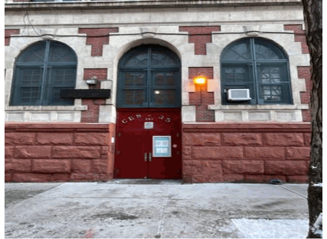
Facade A - North View
