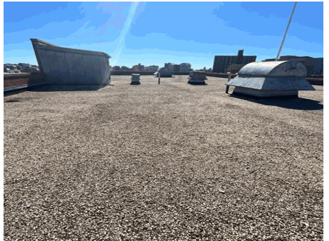
Roof 1 - East View
