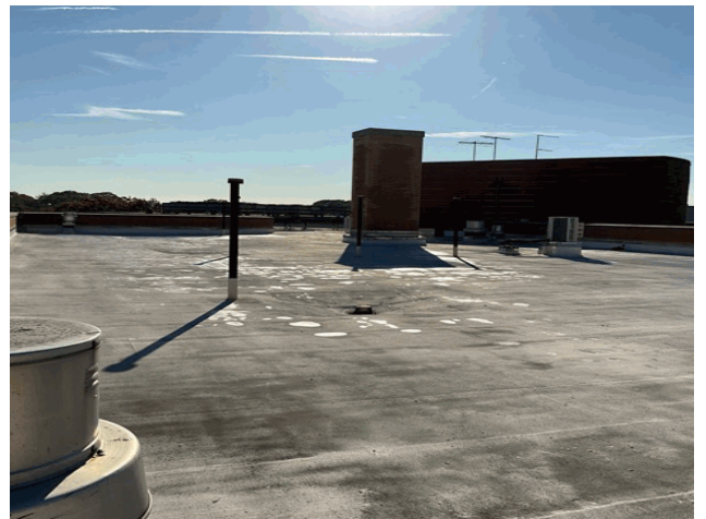
Roof 1 - Southeast View
