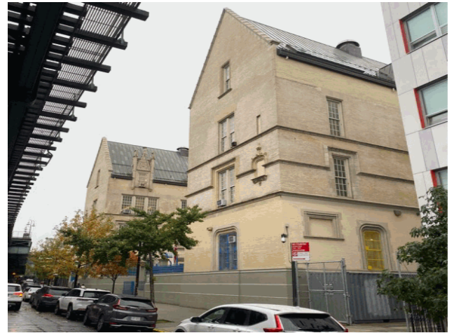
Jerome Avenue - Northeast view
