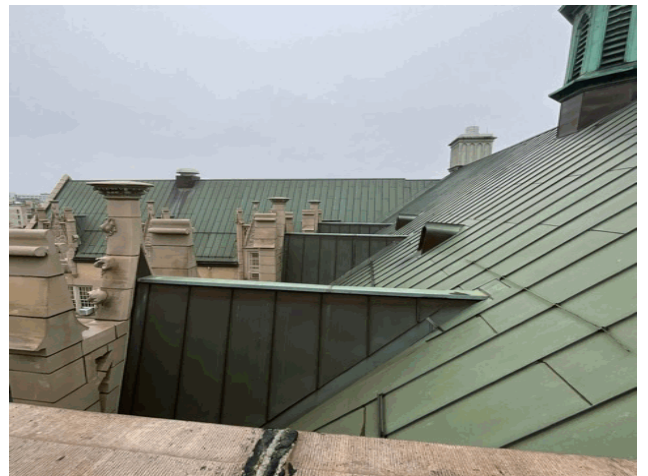
Roof 2 - North view
