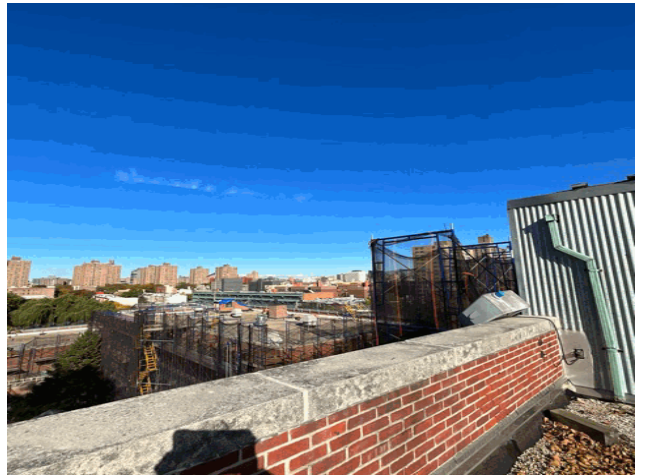
Roof 5 - Northwest View
