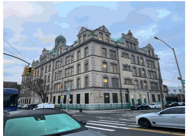
Corner of St. Ann's Avenue and East 148th Street - Southwest View
