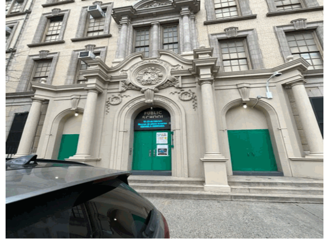
Facade A - St. Ann's Avenue
