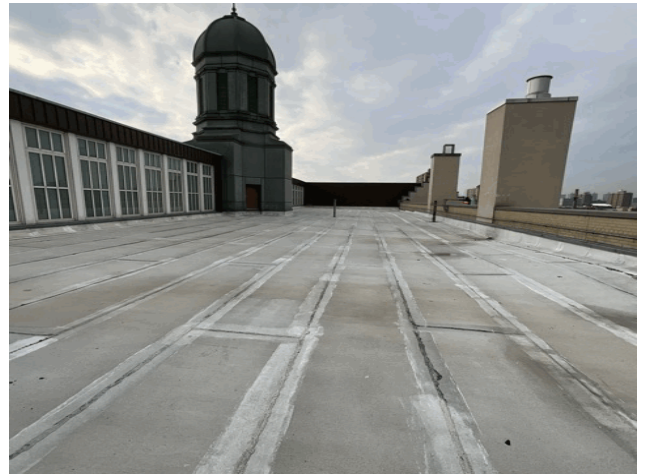
Roof 1 - Southwest View
