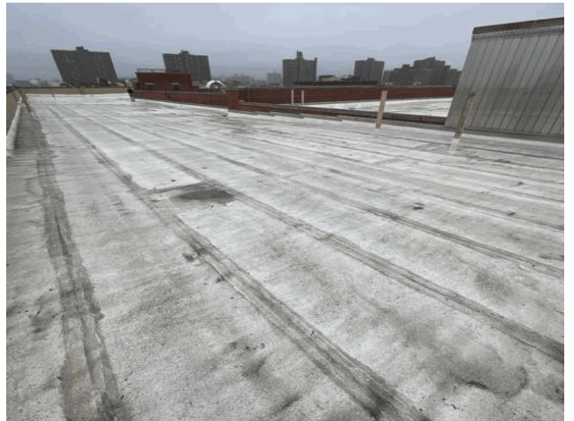
Roof 1 - West View
