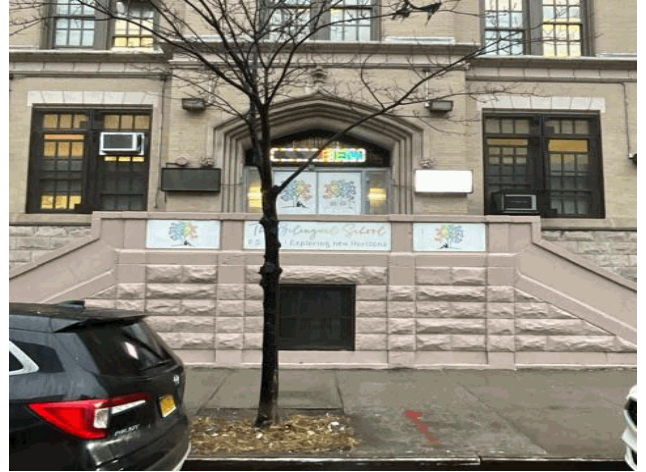
Facade A - East 149th Street
