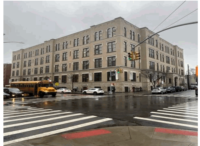
Corner of East 149th Street and Union Avenue - Northwest View
