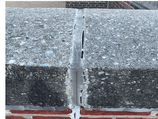
Roof 1 at Facade F
