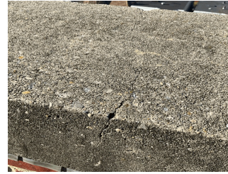
Roof 1 at Facade F
