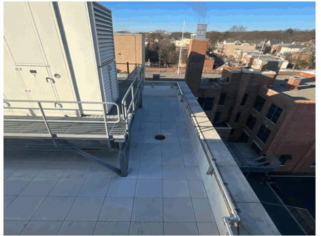
Roof 7 - West view
