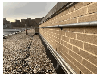
Roof 1 - Facade A
