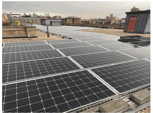
Roof 1 - North view
