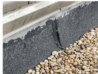
Roof 1 - Facade B
