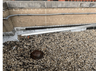
Roof 1 - Facade A
