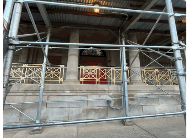
Facade A - Carpenter Avenue
