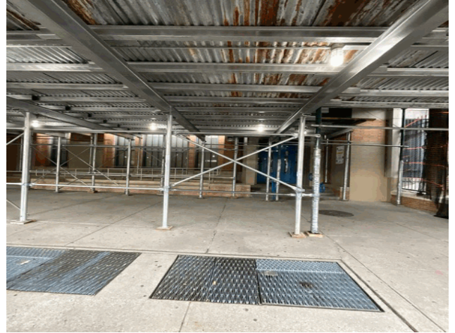
Facade A - Andrews Avenue
