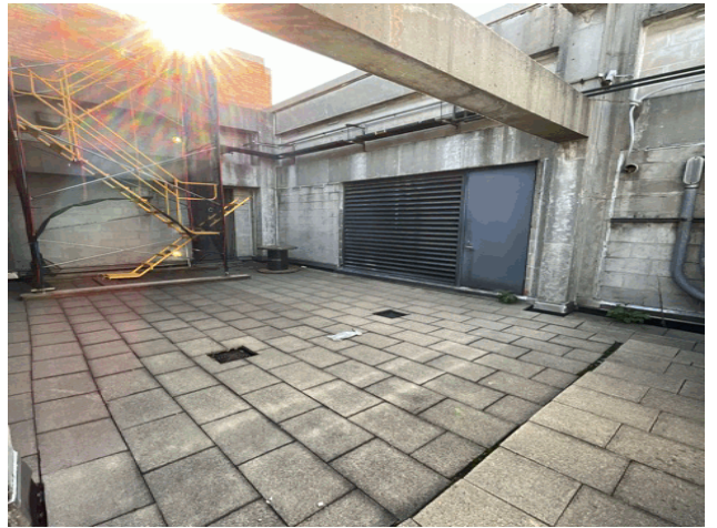
Roof 16 - West View
