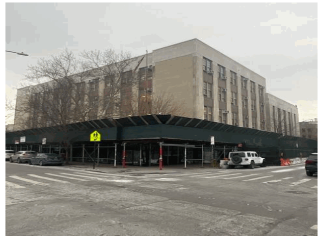
Corner of Ryer Avenue and East 183rd Street - Southeast View
