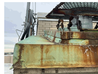
Roof 1 - Skylight SK
