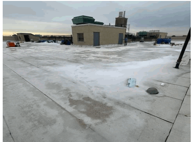
Roof 1 - Southwest View
