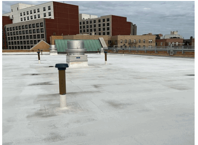
Roof 3 - Northwest View
