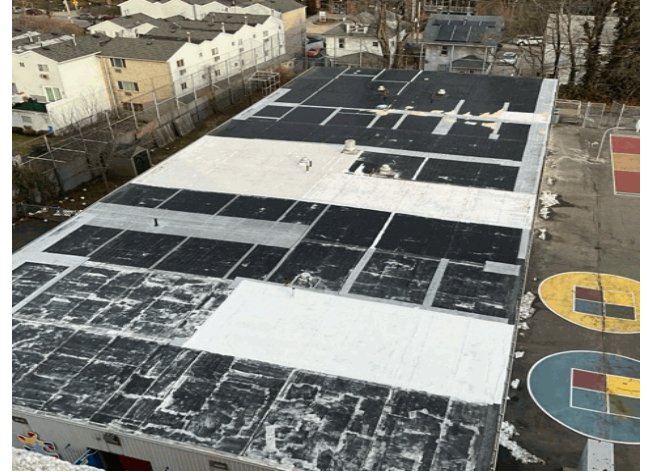
Roof 1 - North View from Main Asset
