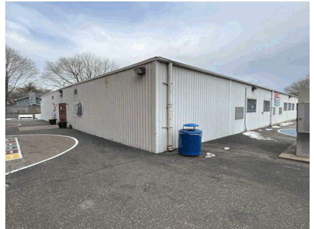
Facades A and D - North View
