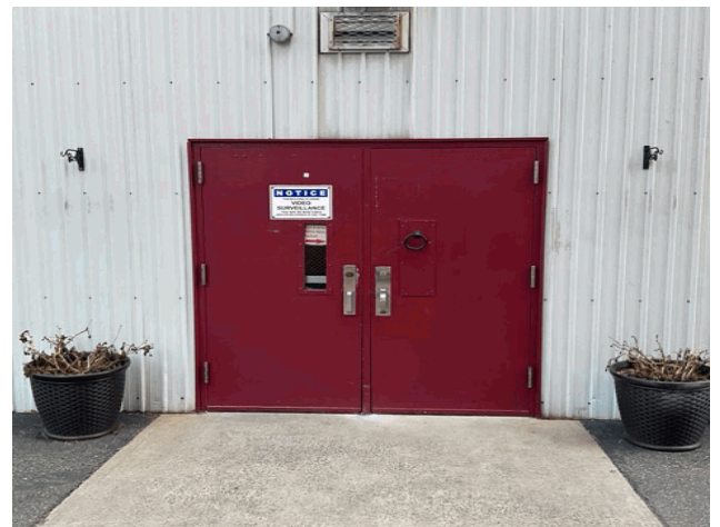
Facade A - Parking Area
