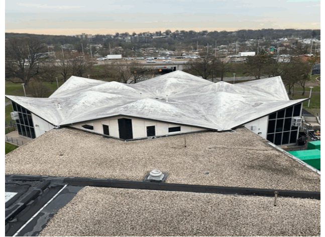
Roof 1 - North View from Asset R886
