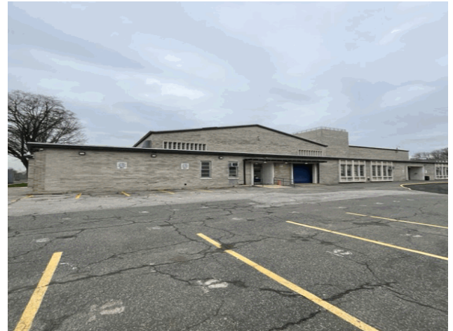
Safety City Boulevard - Northeast View
