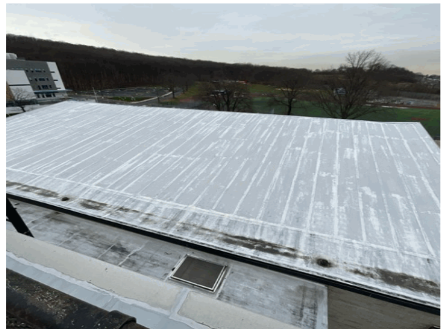
Roof 2 - West View from Asset R886
