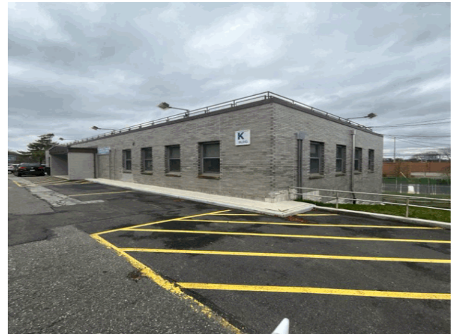
Parking Area - Northeast View
