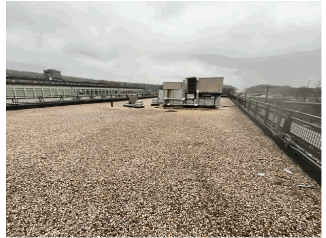
Roof 1 - West View
