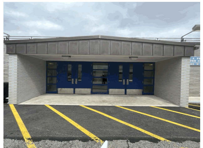
Facade A - Parking Area
