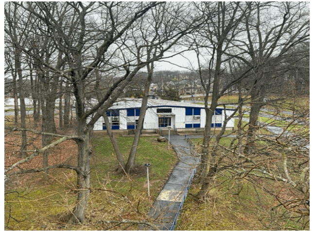
Roof 1 - East View (from R080)
