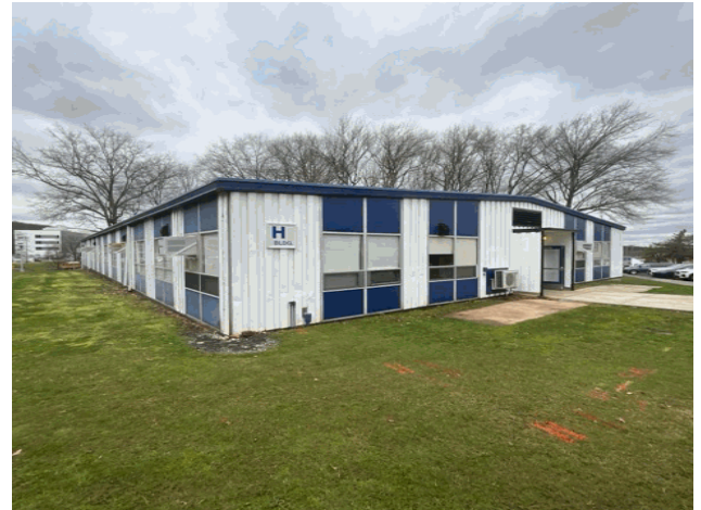
Safety City Boulevard - West View
