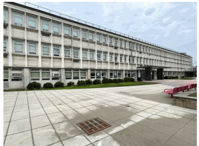
Courtyard/Parking Area - Northeast View
