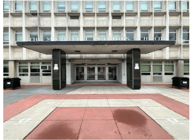
Facade A - Courtyard/Parking Area
