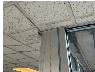
Corridor near Exit W2
