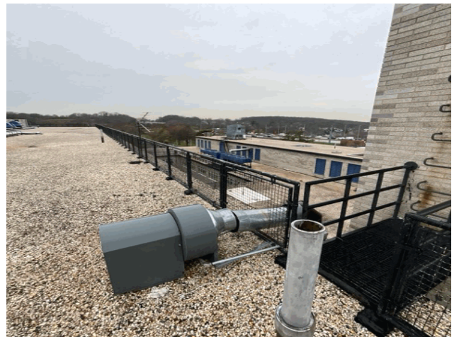
Roof 1 - Northwest View
