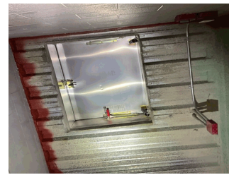
Stair D/2 shown (around Roof Hatch)
