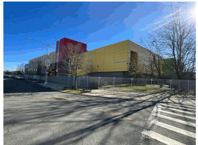
Corner of Regis Drive and Farragut Avenue - Southwest View
