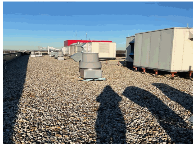
Roof 1 - Northwest View
