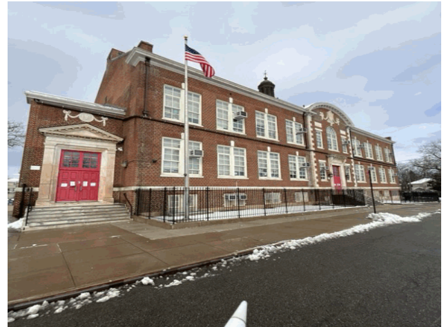
Augusta Avenue - Northeast View
