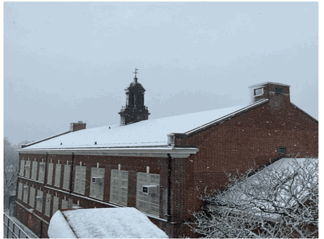
Roof 1 - West View
