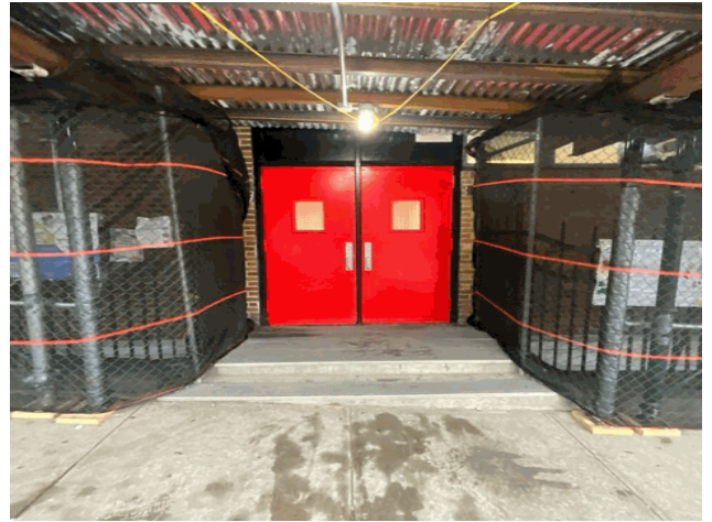
Facade A - Daniel Low Terrace
