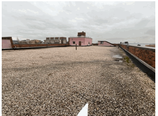
Roof 1 - North View
