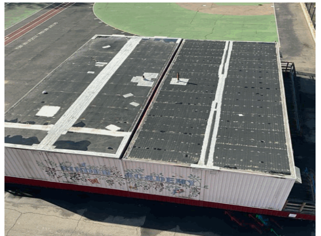
Roof 1 (from main asset)
