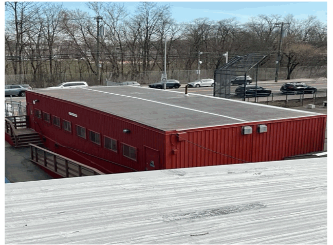
Roof 1 - East View from Main Asset R038
