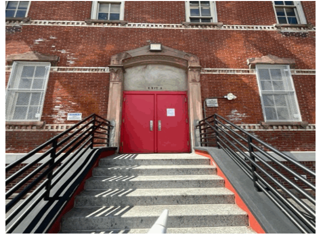
Facade A - Yetman Avenue
