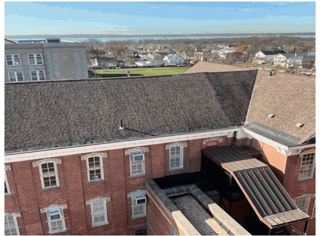
Roof 1 - South View from Main Asset R001
