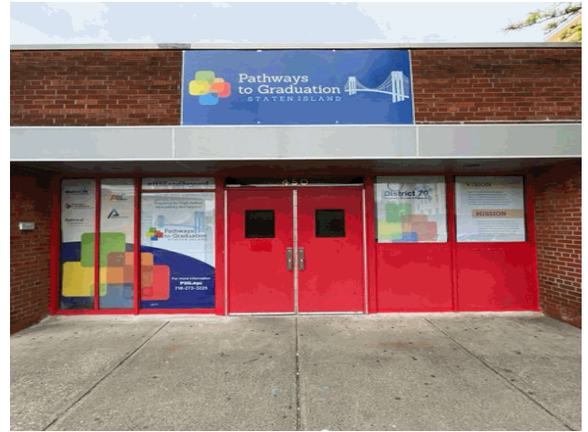
Facade A - St. Marks Place
