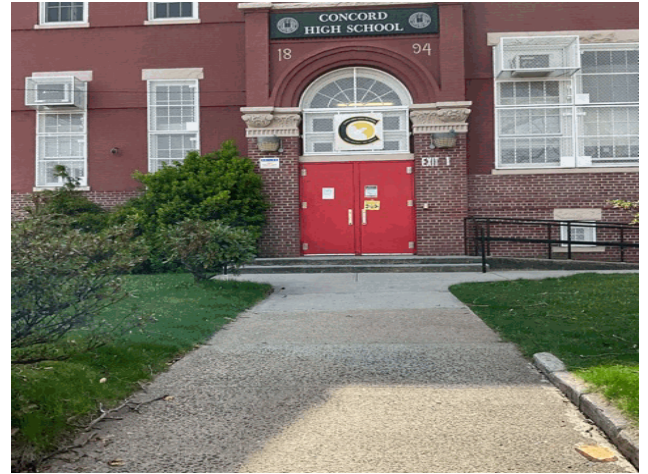
Facade A - Rhine Avenue
