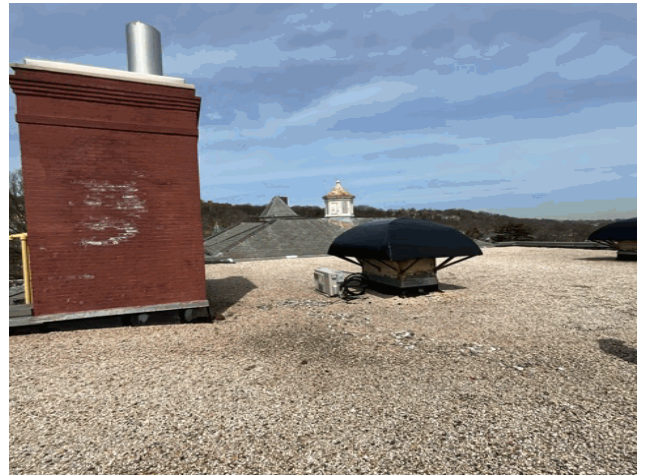
Roof 3 - North View
