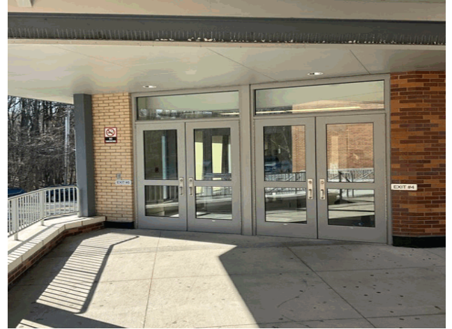
Facade A - Manor Road
