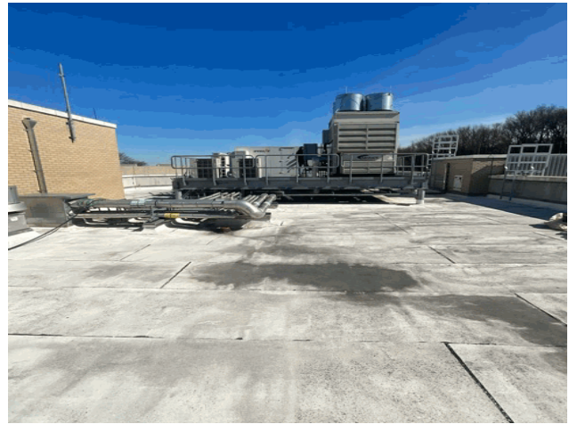
Roof 2 - South View
