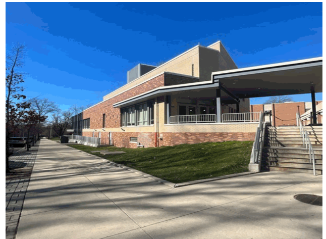
Manor Road - Southwest View
