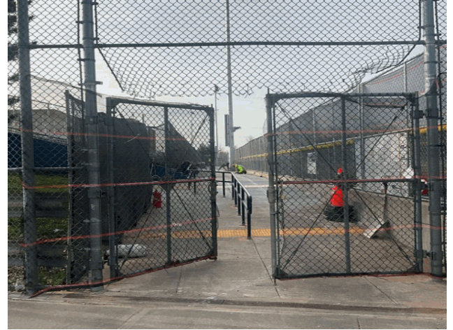
Brielle Avenue - Main Entrance
